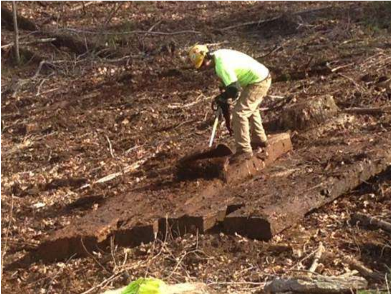
Cleaning Swamp Mats with Power Broom During Forestry Operations
