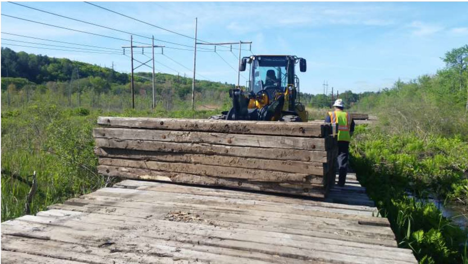
Stacking swamp mats to be brought to designated cleaning area
