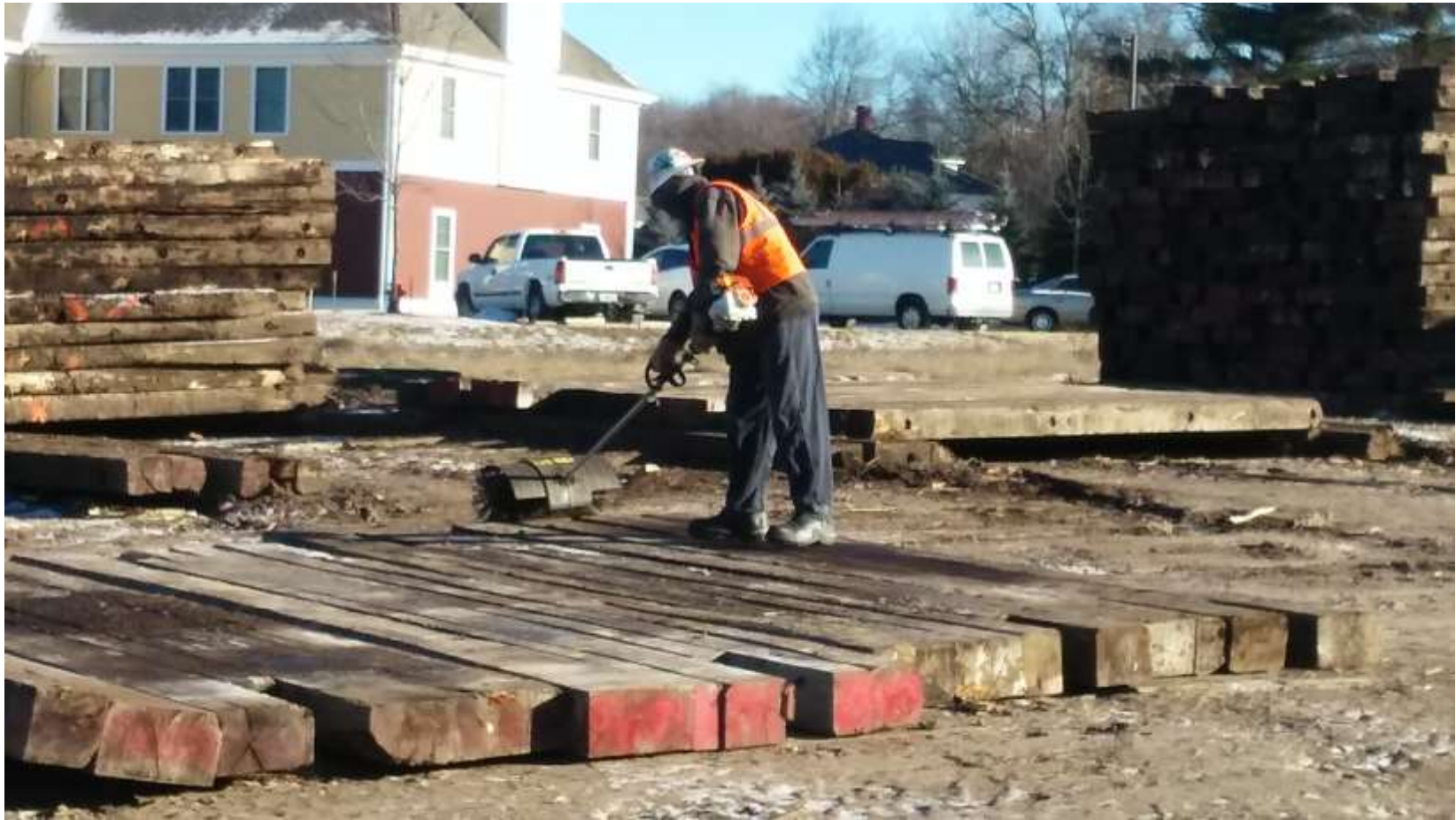
Cleaning Swamp Mats with Power Broom in Upland Staging Area
