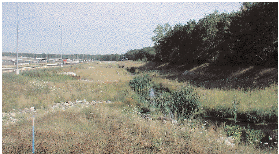
The evolution of a river. Depicted from top to bottom: preconstruction condition, April 2001; stabilization of the newly excavated river corridor, June 2001; and the corridor after substantial vegetation establishment (despite drought), August 2002.
