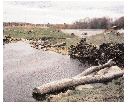
Interplanted with wetland grasses and forbs, channel edges, left, are secured with rounded gravel, irregularly sized riprap and coir rolls. Live cuttings from native shrubs sprout along the banks. Right, woody revetments—such as fallen tree shelters and root wads recovered from the stadium site construction—immediately stabilized channel and pool edges prior to vegetation establishment. The flood-control access berm is in the background.
