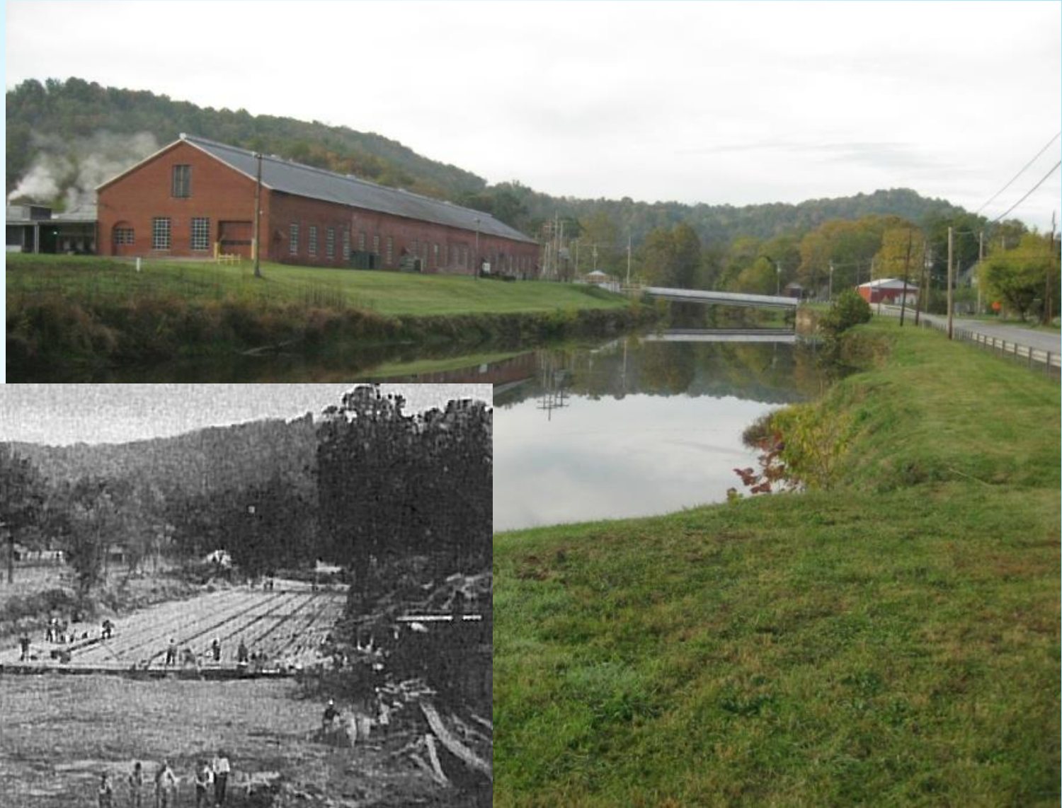
Cooling Pipes for Gas Pumping Station Under impoundment
