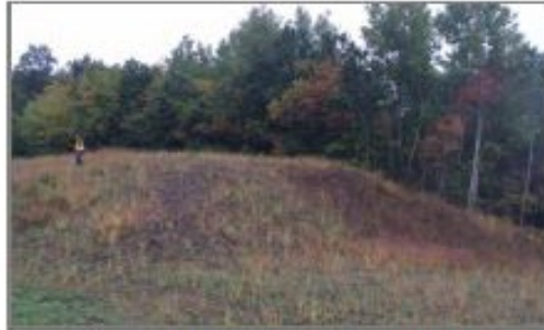
Slopes prior to application, Sept. 21st
